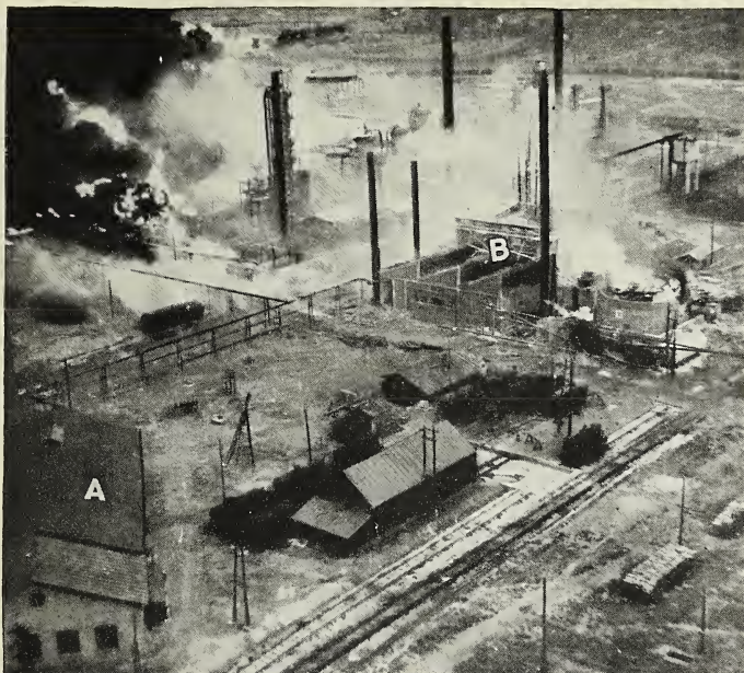
A portion of the flaming Colombia refinery, showing the boiler house (A) and power house (B).
